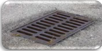
Stormwater drains prevent flooding by allowing rain water to run off of impervious surfaces (for example: concrete) and into natural water bodies (for example canals).
