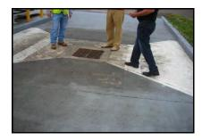
Visual inspections of the drainage conveyance system structures are conducted semi-annually, or every 36 months, to make sure the system is operating correctly and free of obstruction. Should a structure be obstructed or fail, measures are taken to clear or repair the structure.
