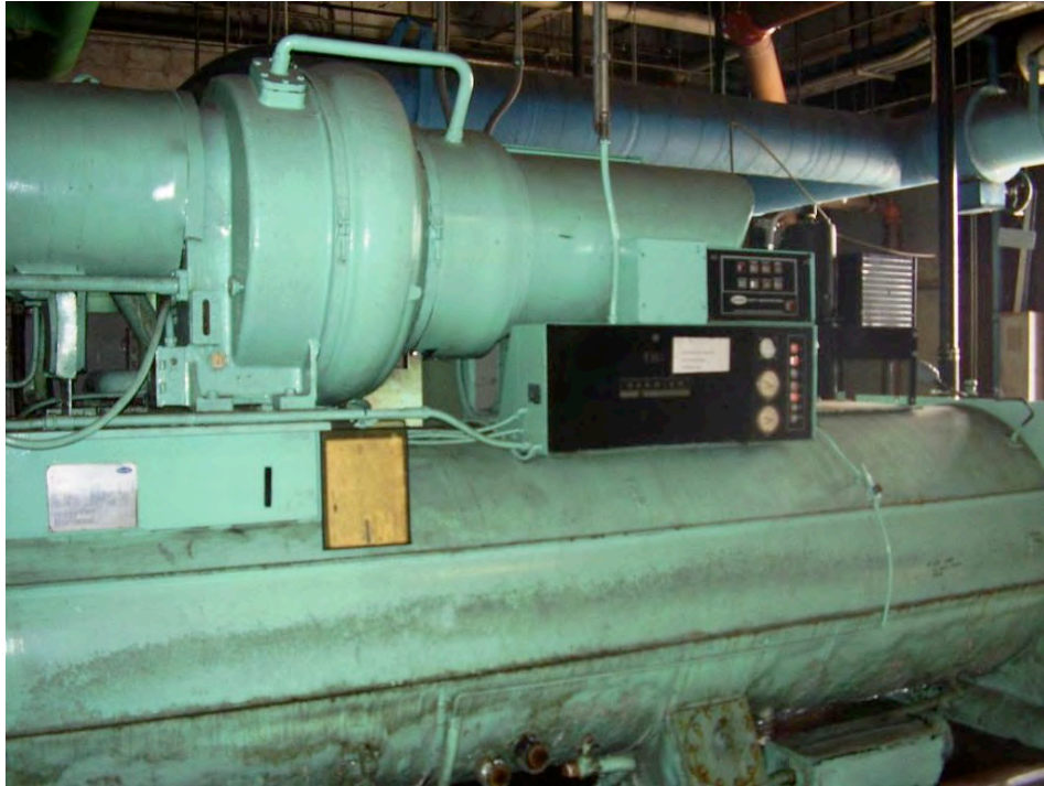
Existing Carrier Chiller in Terminal 4
