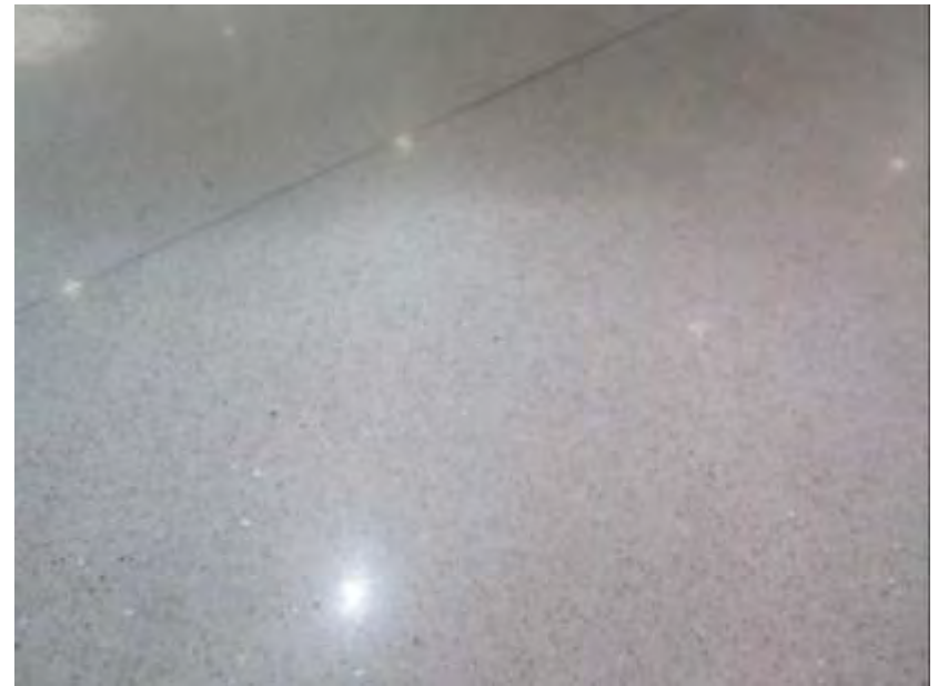
Figure 31: Newly Installed Terrazzo Floor Standard at FLL Terminal 3
