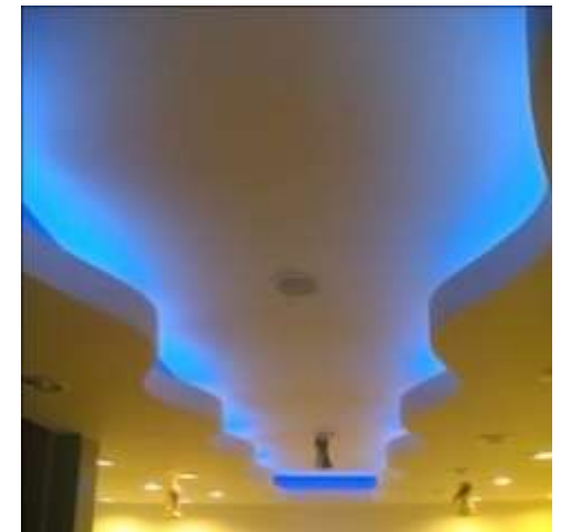
Figure 50: Example of cove ceiling lighting
