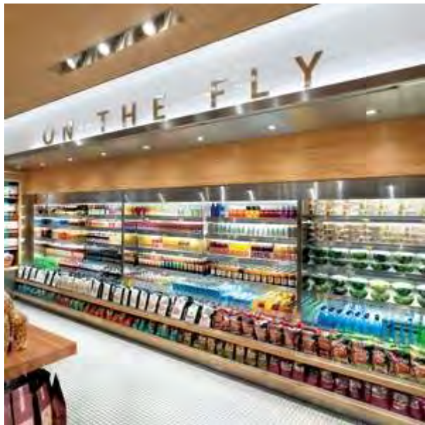
Figure 35: Example of Integrated cooler with wall finishes
