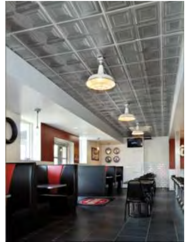
Figure 48: Example of simple Tenant lighting fixtures
