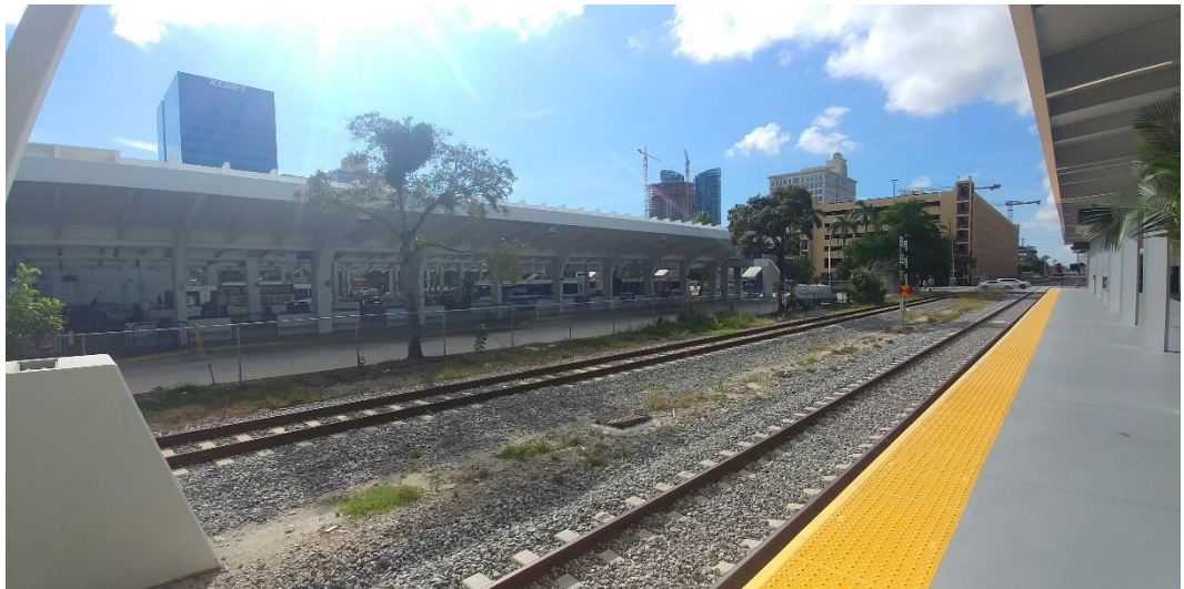
Existing condition photo of the fence looking eastbound from Brightline Station
