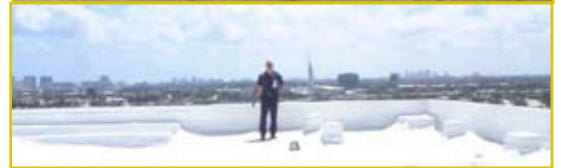
Temperature readings taken on conventional roofing compared to the new Spray Polyurethane roofing show a 39 degree difference.
