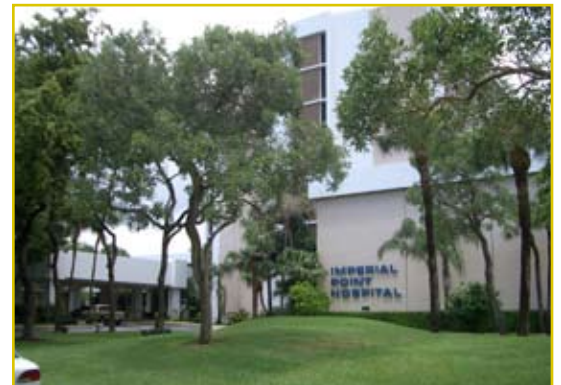
Hospital grounds reflect good coverage by the irrigation system using the energy management system.
