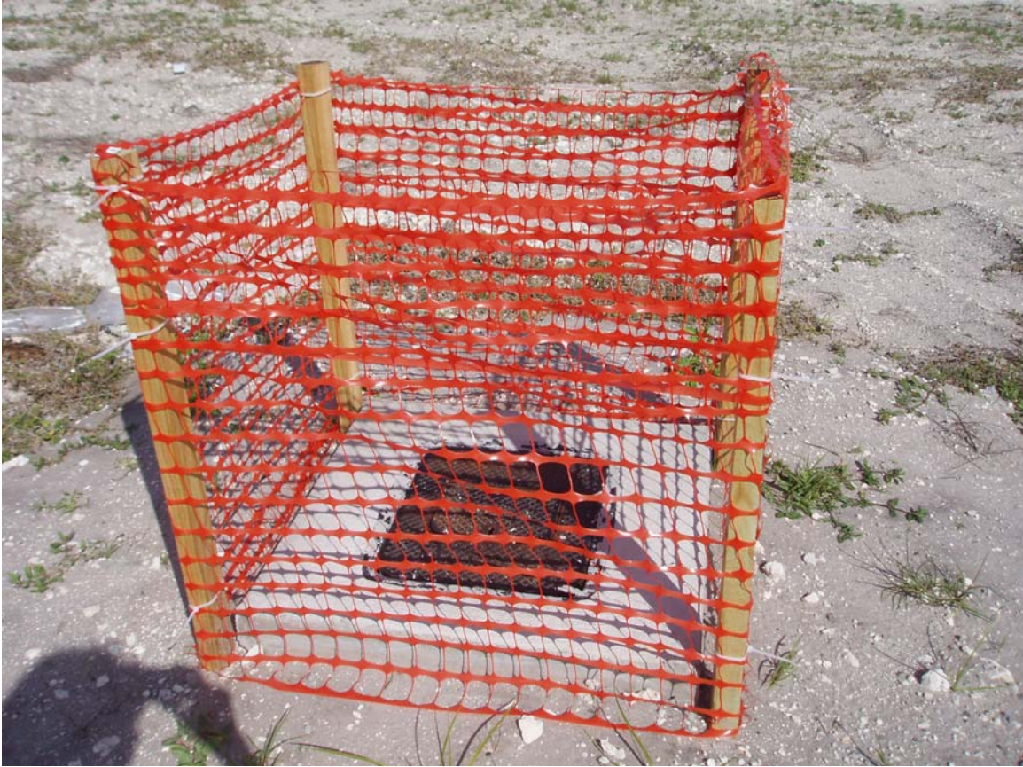
Picture 1 – Secured Water Service at Finished Grade
