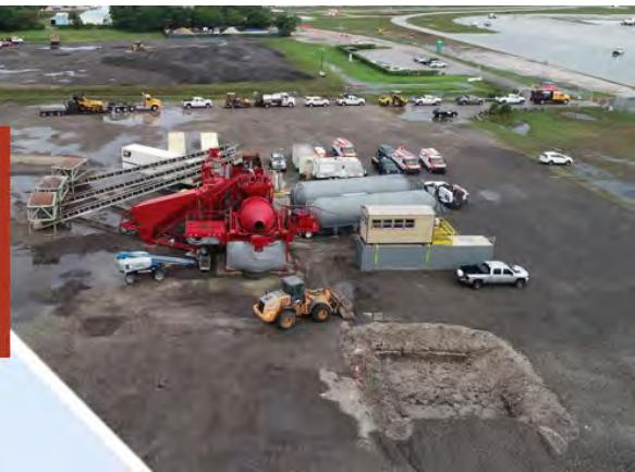
The North Runway, (10L-28R), the oldest of FLL's two runways, is undergoing significant rehabilitation and was closed temporarily on June 3, 2019, for up to four months. The critical rehabilitation work will include replacing the runway's 75-foot center portion with concrete to extend its life from 15 to 30 years and repaving of its sides with asphalt.
