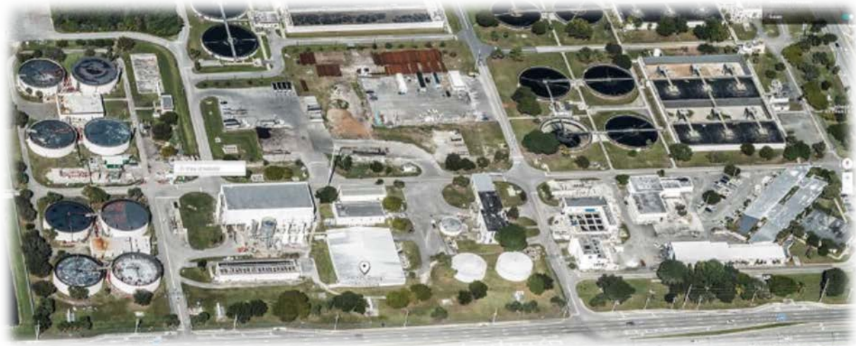
Figure 1: Water and Wastewater Treatment Facility
