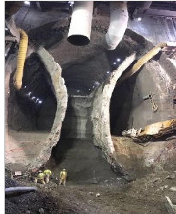
Figure 32: Construction During SEM Example 4
