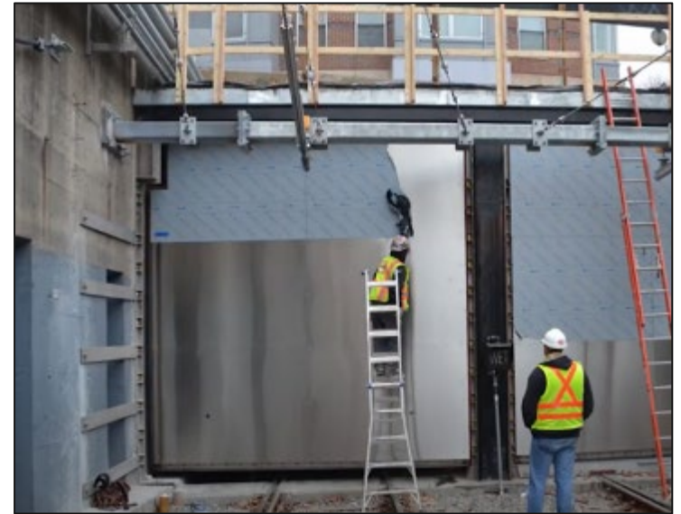
Figure 35: Floodgates Installation
