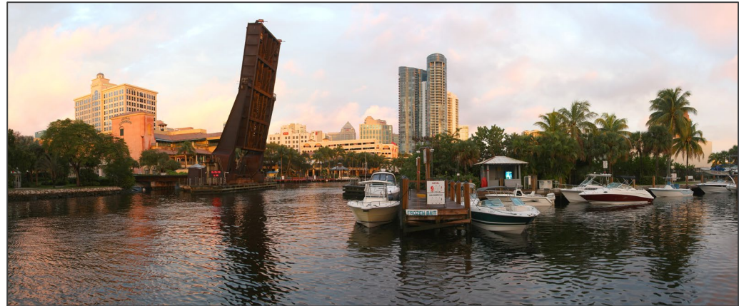
Figure 1: Bascule bridge on New River
