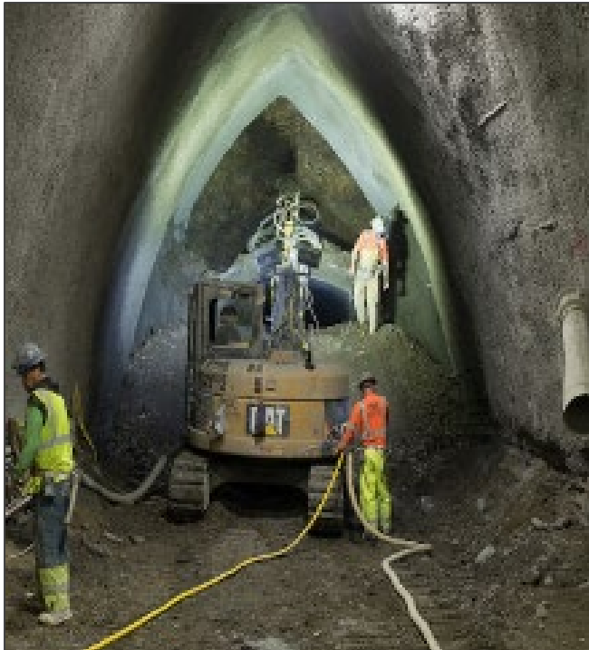
Figure 33: Construction During SEM Example 3
