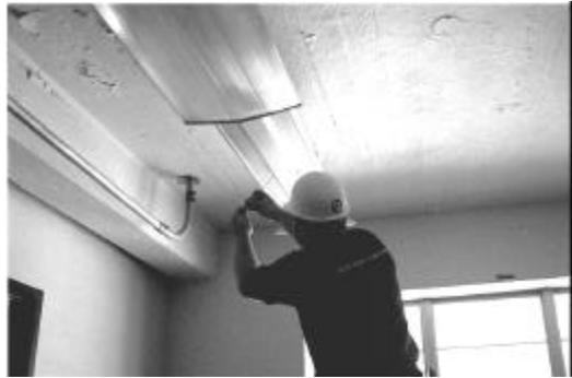
After removing bulb, remove ballast cover.
