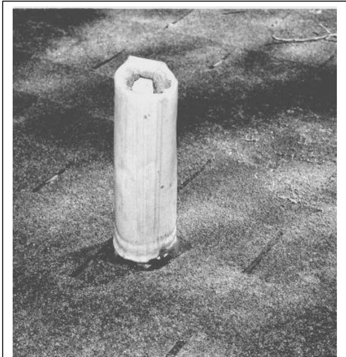
The durable and malleable properties of lead make it an excellent material for protecting and sealing pipes and vents on roofs.
