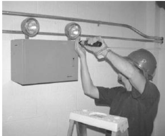
*Remove Panel Door Fasteners*
