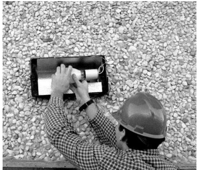
HID Bulb may be removed by unscrewing from fixture.
