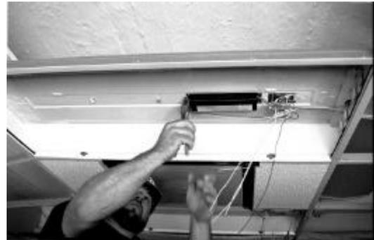
Cut wires and remove ballast.
