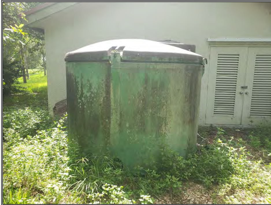
Above: A representative view of the one (1) approximately 1,000-gallon high-density polyethylene (HDPE) aboveground storage tank (AST) containing liquid fertilizer on the second parcel of the Subject Property observed during the site reconnaissance.
