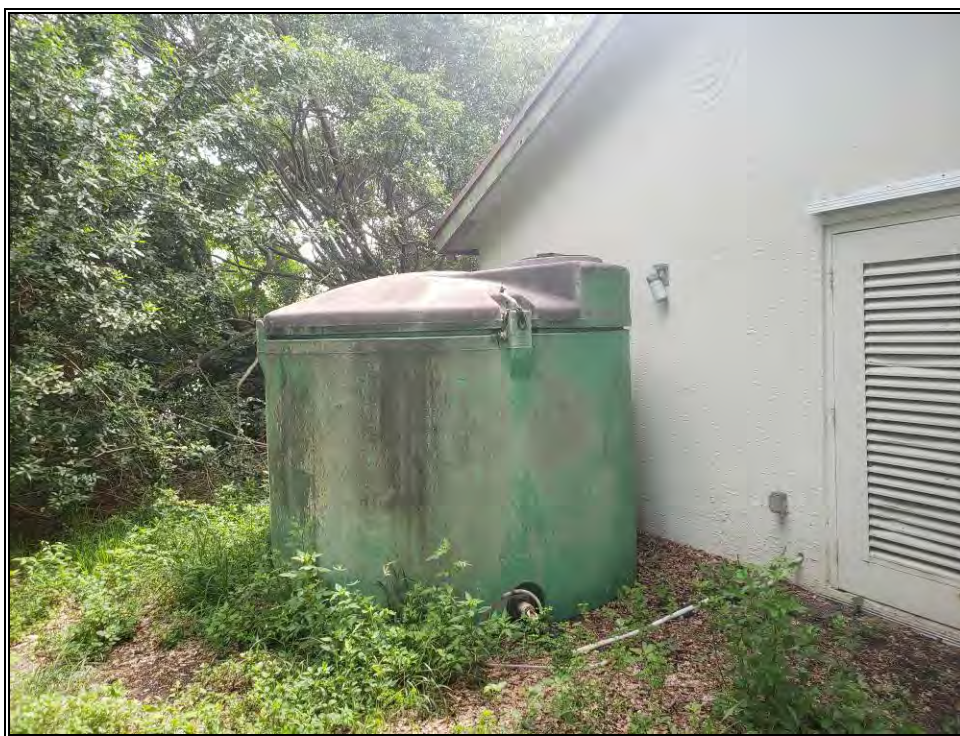
Above: A representative view of the one (1) approximately 1,000-gallon HDPE AST containing liquid fertilizer on the second parcel of the Subject Property observed during the site reconnaissance.
