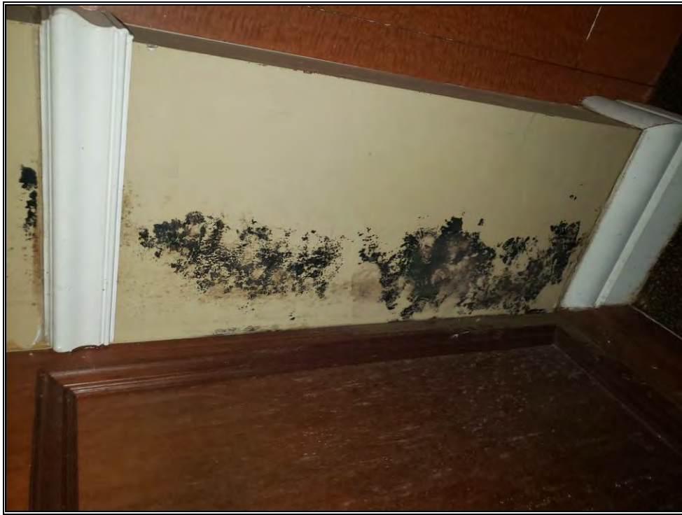
Above: A representative view of mold in the interior of the commercial structure on the fourth parcel of the Subject Property observed during the site reconnaissance.
