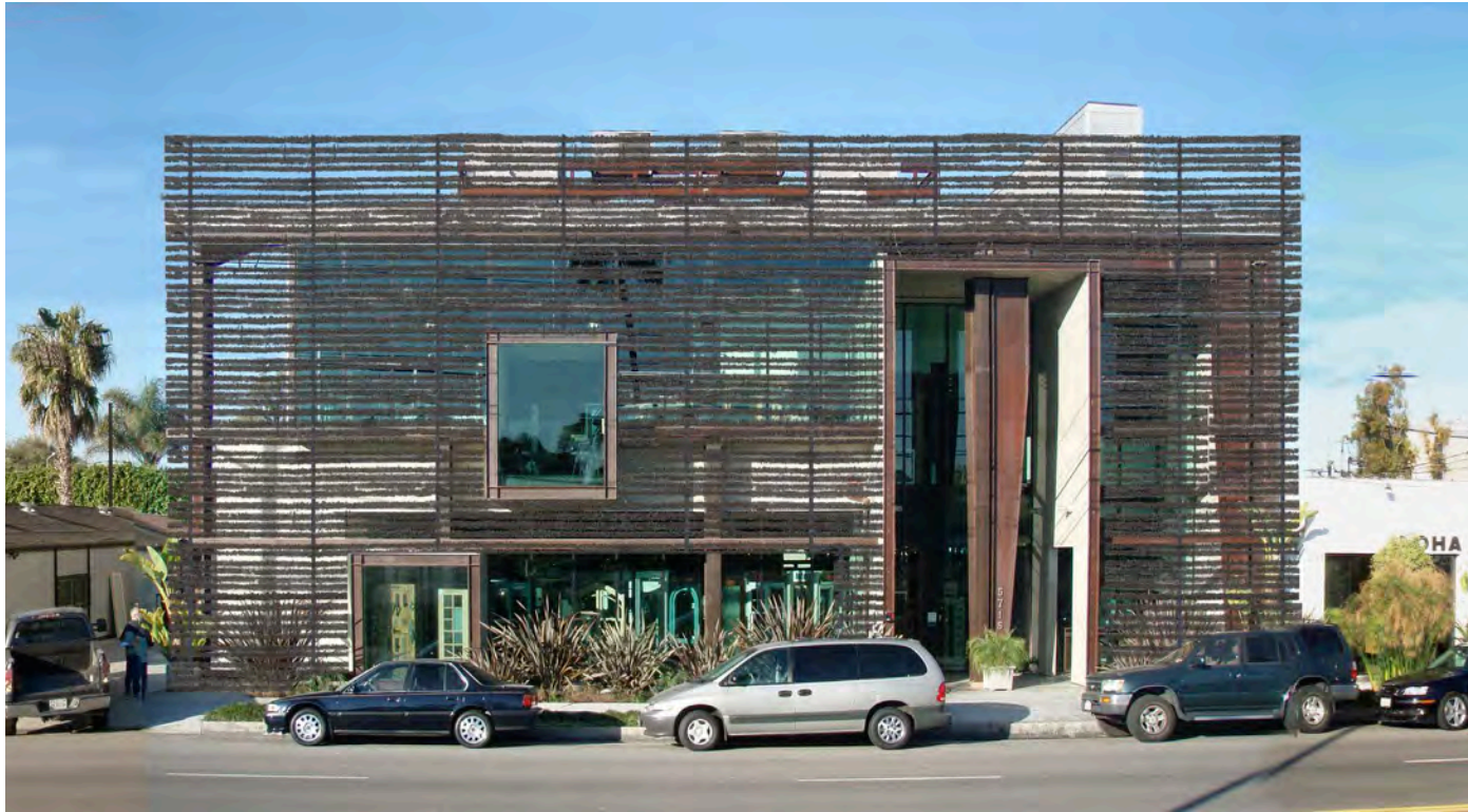
View of the main street entry showing the facade made from industrial broom technology..
