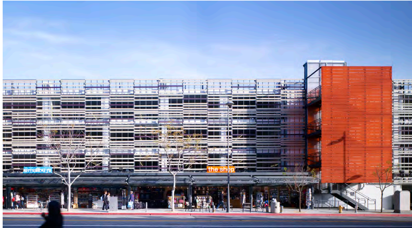
View from Broadway St. showing the new facade and retail added to the ground level.
