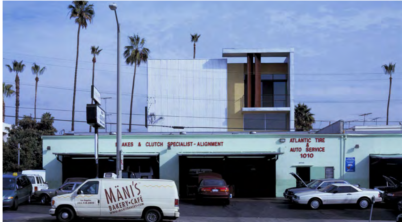
View from Fairfax Blvd.
