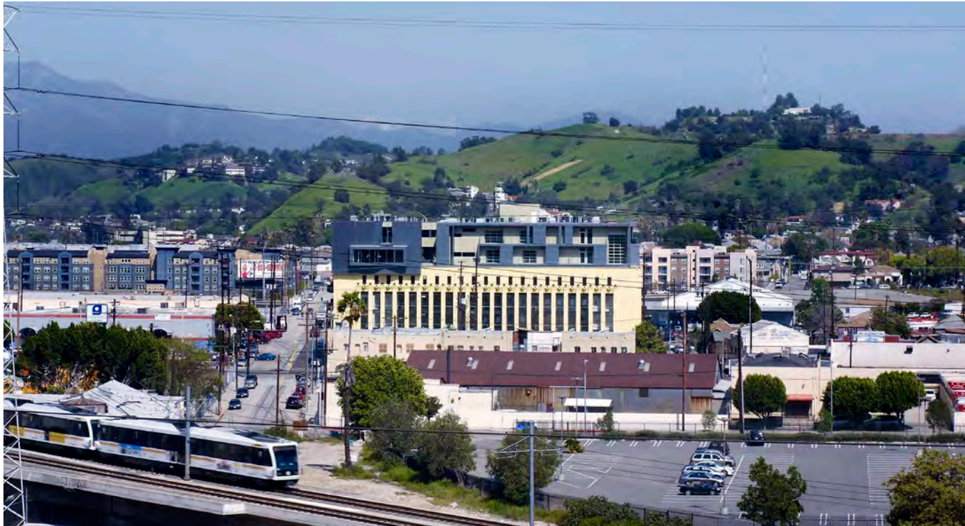
View of the new addition on top of the historic 1920 concrete warehouse built for the Fuller Paint Company.
