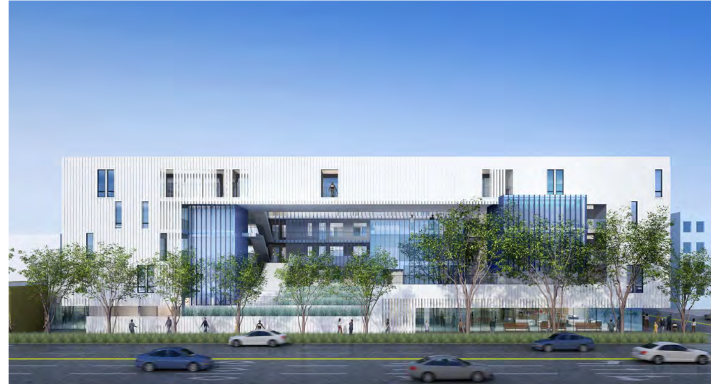
Main building facade along Camarillo Ave (above). Backman Street (below).
