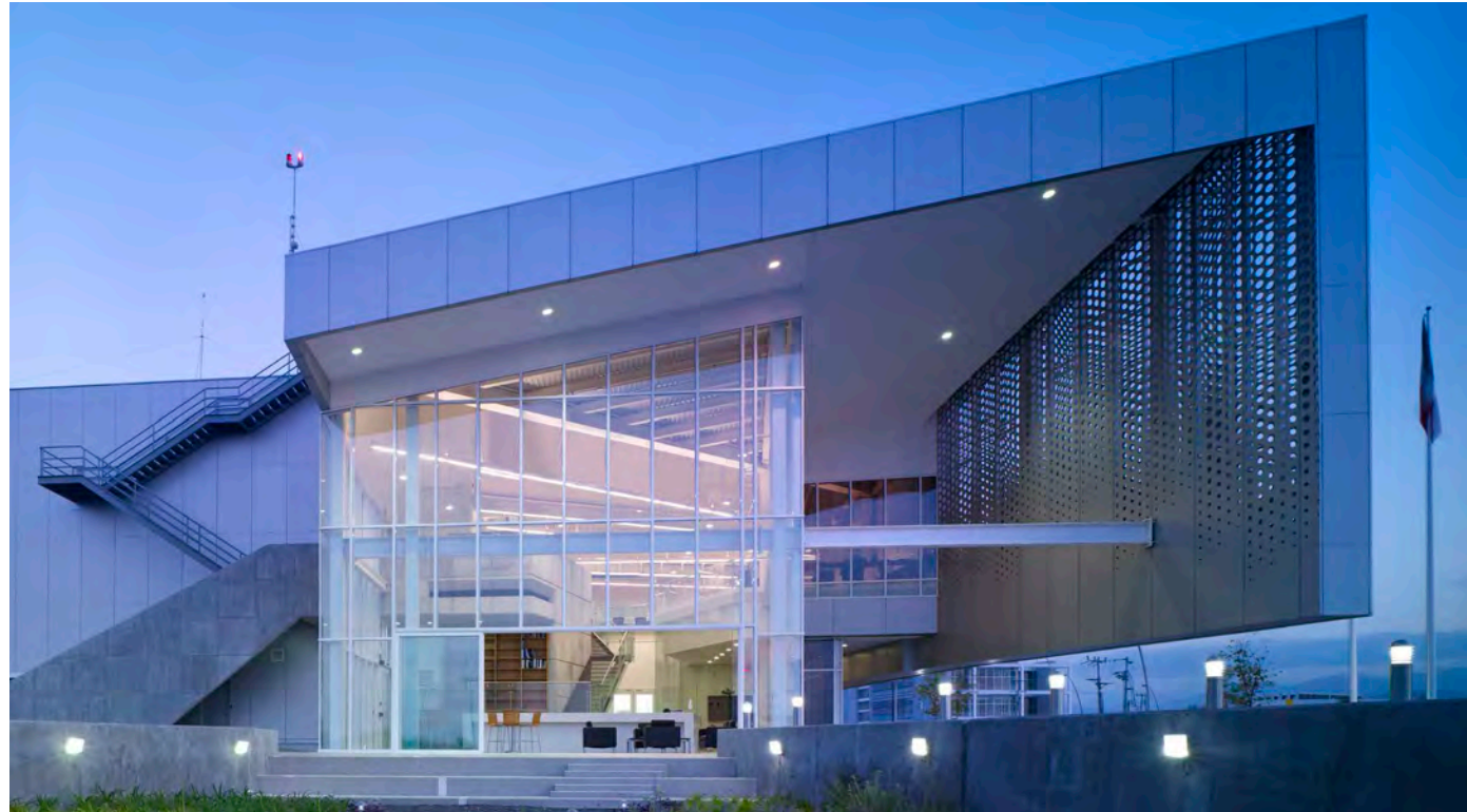
View from the garden looking at the north facade towards the lobby and main entry.
