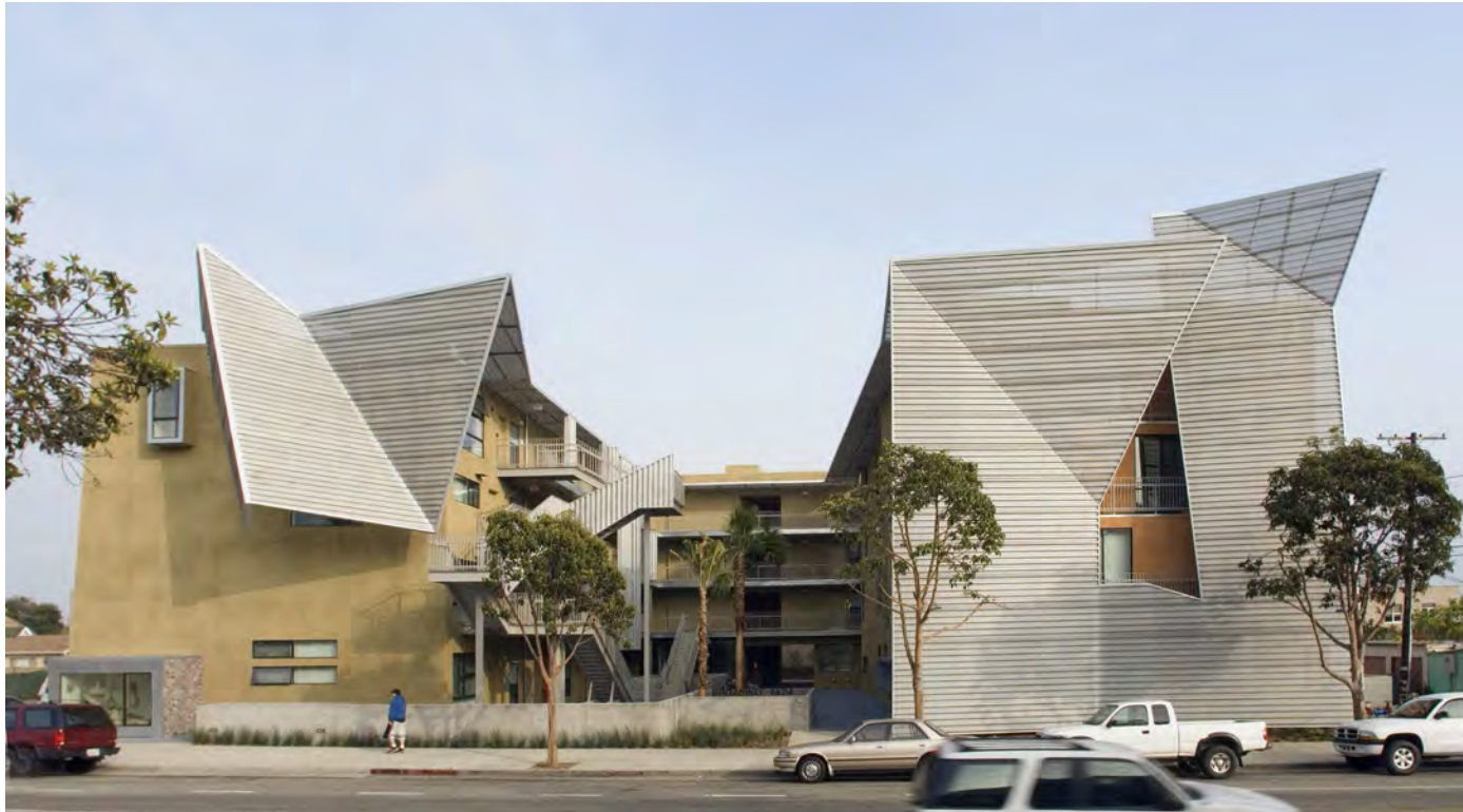
View of the entry courtyard from Broadway showing the perforated aluminum shade screens and facade..
