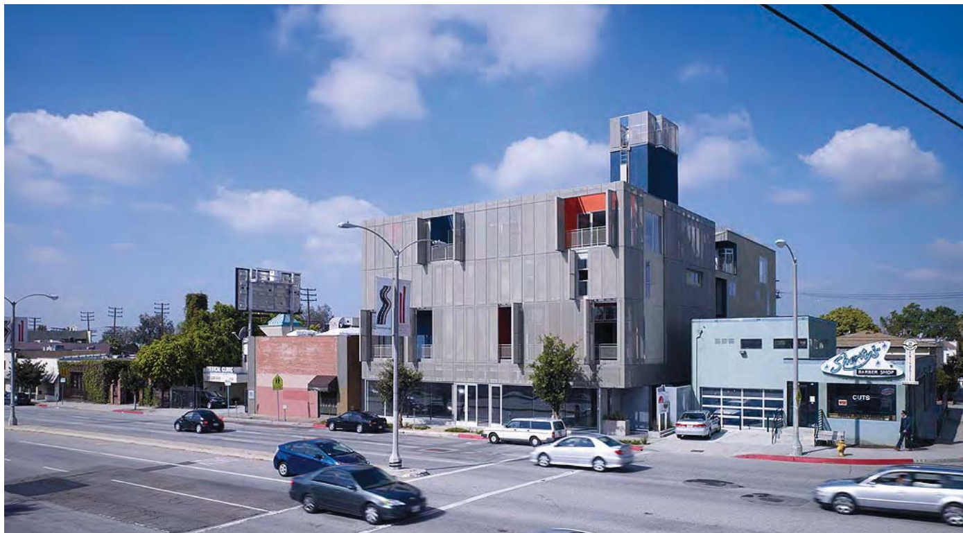
View from Fairfax showing the prefabricated operable aluminum screens.
