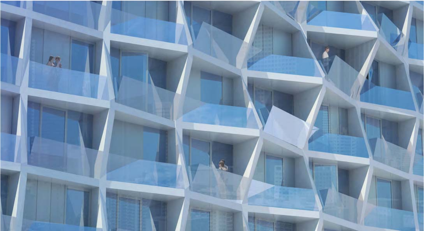
Detail view of the facade and alternating balcony system.
