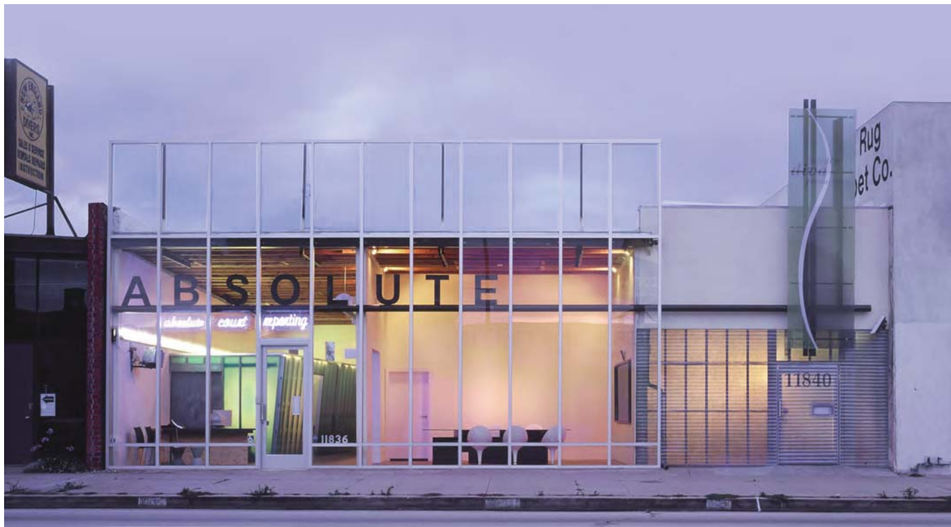
Remodeled facade along Pico Blvd (above). Facade detail (opposite). Before remodel (insert).
