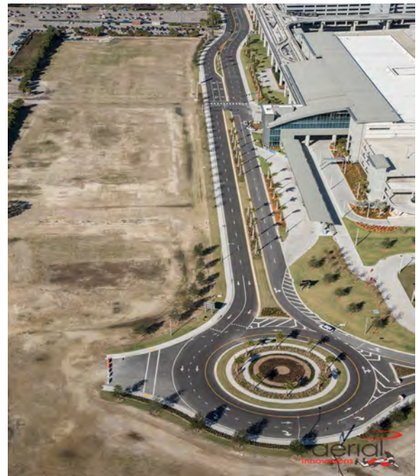
Tampa Airport roadway improvements.
