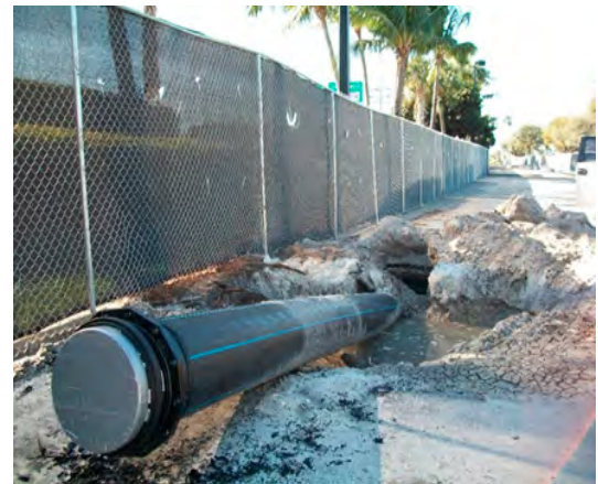
Construction inspections at Seminole Hard Rock Hotel and Casino.
