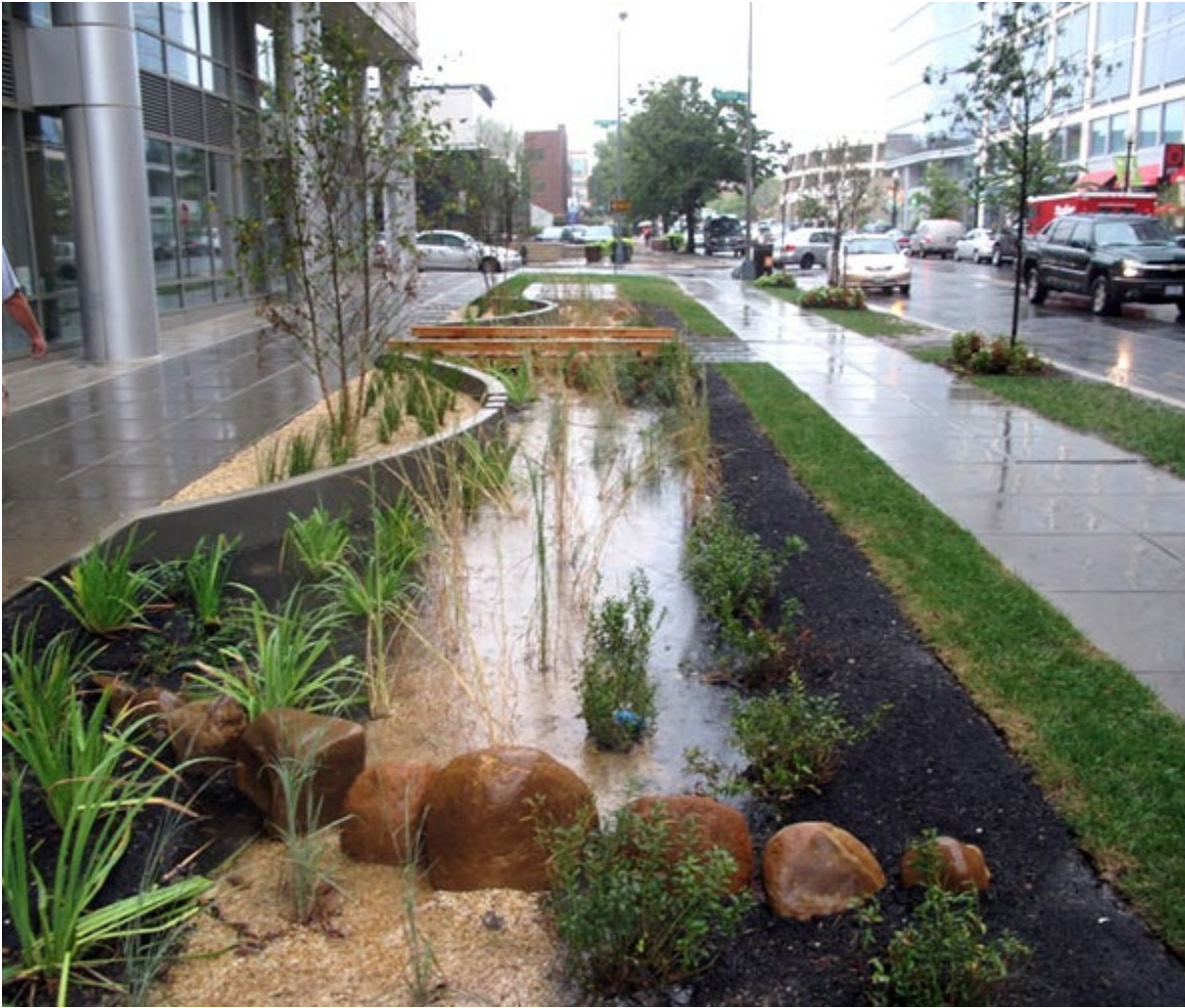
Rain gardens are a form of green infrastructure incorporated into sidewalk design in Washington, DC.
