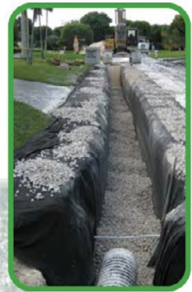
Exfiltration Trench Systems
