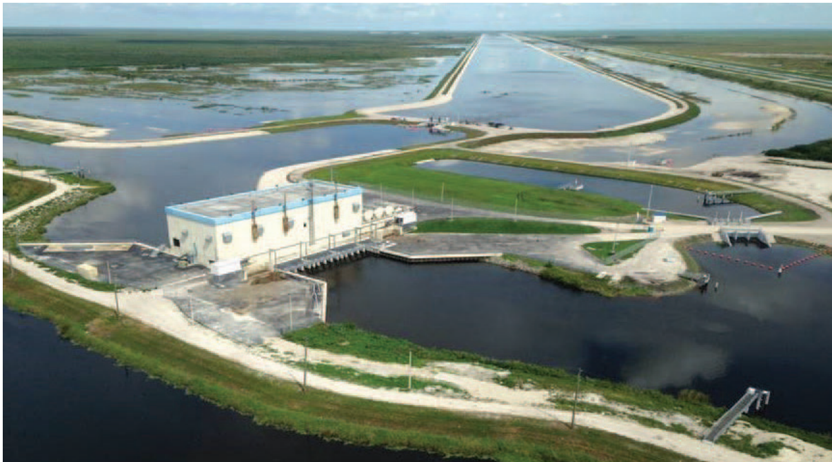
A flow equalization basin - or FEB - is a reservoir designed to temporarily capture and hold stormwater runoff for release to the Everglades stormwater treatment areas (STAs). By tempering flow rate, FEBs help maintain desired water levels in the STA. The A-1 Flow Equalization Basin (pictured above), just north of the Broward County line along US Highway 27, is part of Florida's Restoration Strategies Plan for clean water for the Everglades, and assists in optimizing the performance of two nearby stormwater treatment areas in removing phosphorus. It can hold up to 60,000 acre-feet of water up to 4 feet deep, and then delivers water in a controlled manner to the treatment areas. It is surrounded by 21 miles of levees and has 15 associated water control structures.
