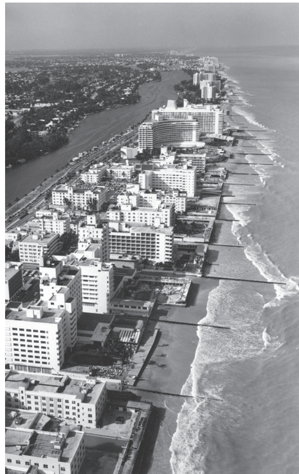
1968 aerial view of the groynes built along Miami Beach near 41st Street. The groynes were built to trap ocean sand filtering south from the Savannah River to maintain a good bathing beach. In reality these structures disrupted the natural flow of sand, robbing beaches downdrift of sand and causing new erosion problems.
