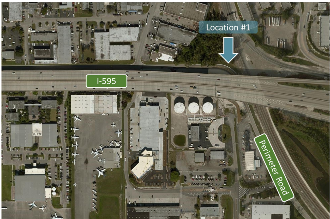
Figure 9: Location #1 - Perimeter Road, Near the I-595 Overpass
