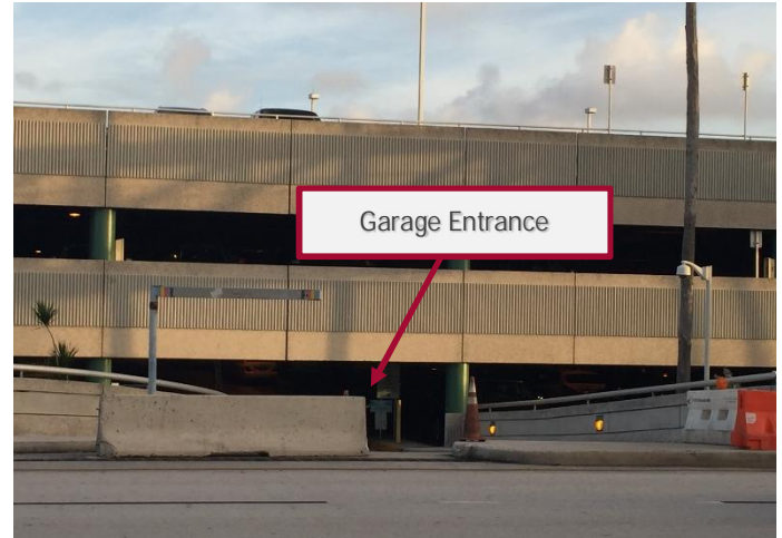
Figure 61: Blocked Garage Entrance
