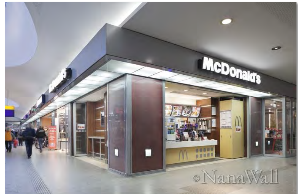
Figure 29: Folding glass door storefront (Notice enclosed pocket at right when open.)
