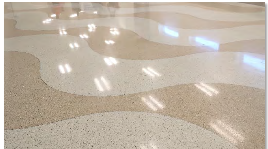
Figure 31: Newly Installed Terrazzo Floor Standard at FLL Terminal 4
