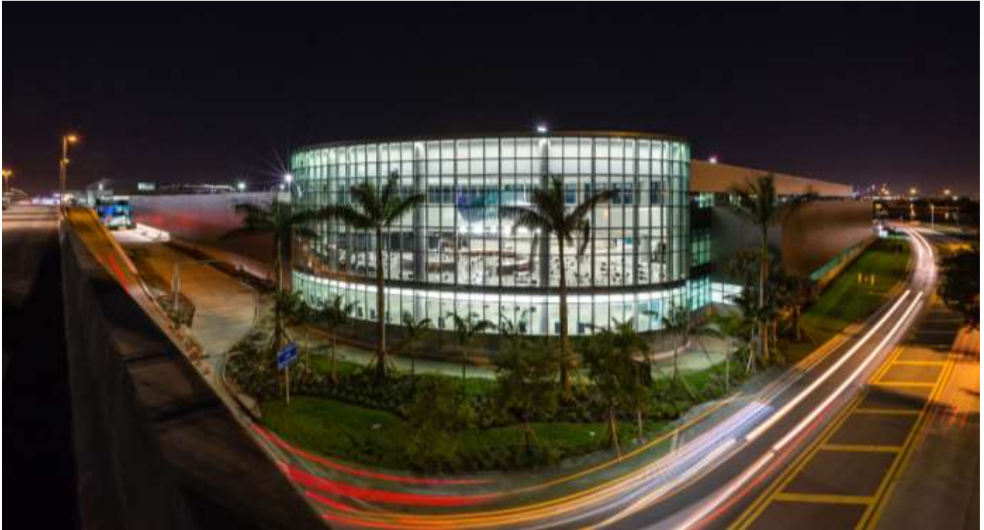
Figure 14: FLL Terminal 1 Concourse A
