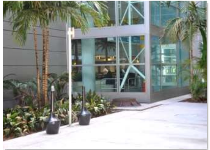
Figure 18: Airport Curtain Wall System at T1 Curbside
