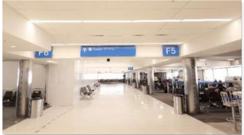
Figure 110: Example of existing FLL Linear Lighting at Terminal 3 Concourse F
