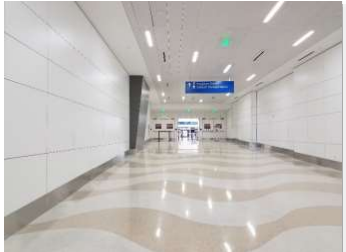
Figure 40: Demounted wall system at FLL T1 Concourse G Exit Corridor
