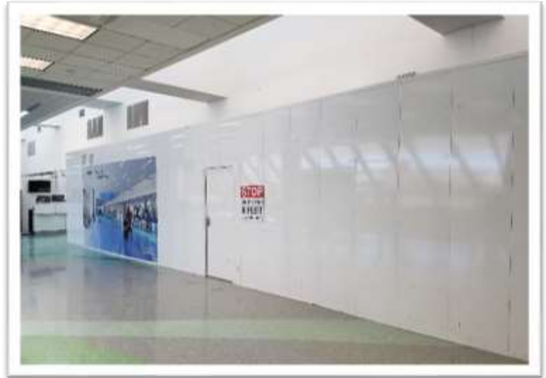
Figure 7: Temporary construction walls “McCain Walls”
