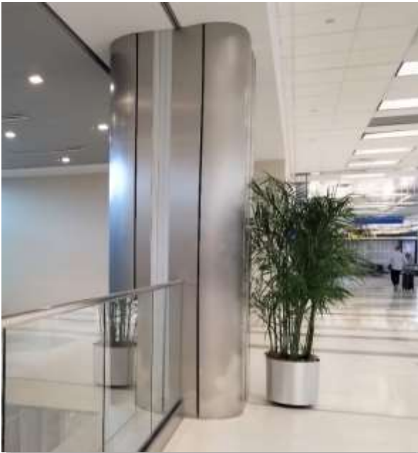
Figure 49: Example of Stainless Steel Column Cover at Terminal 2 Ticketing Level
