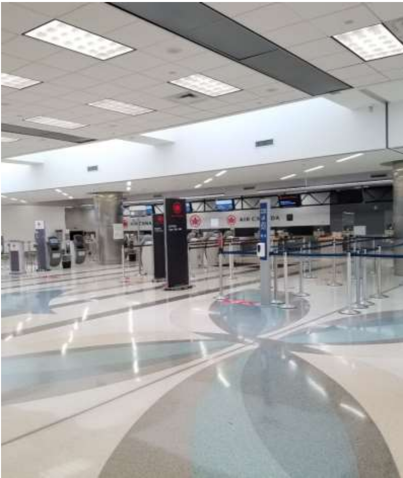
Figure 37: Terrazzo Flooring at FLL Terminal 2
