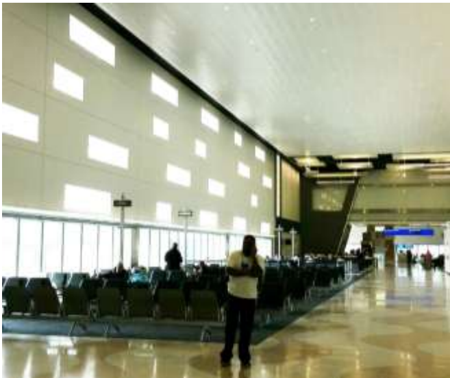
Figure 20: Slot Glazing at FLL, T4 Concourse G
