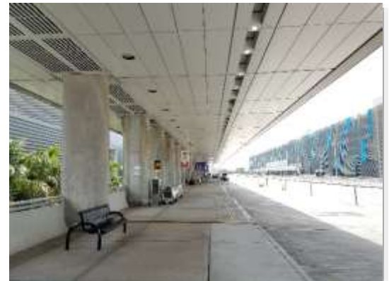
Figure 32: Existing Metal Soffits at FLL Terminal 1
