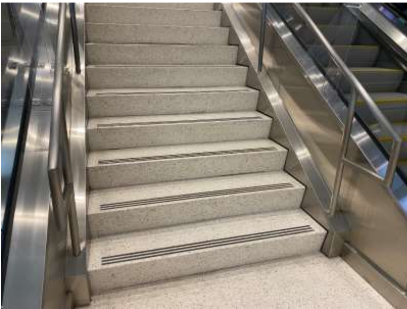
Figure 51: Example of Terrazzo Stairs at Terminal 2 Ticketing Level
