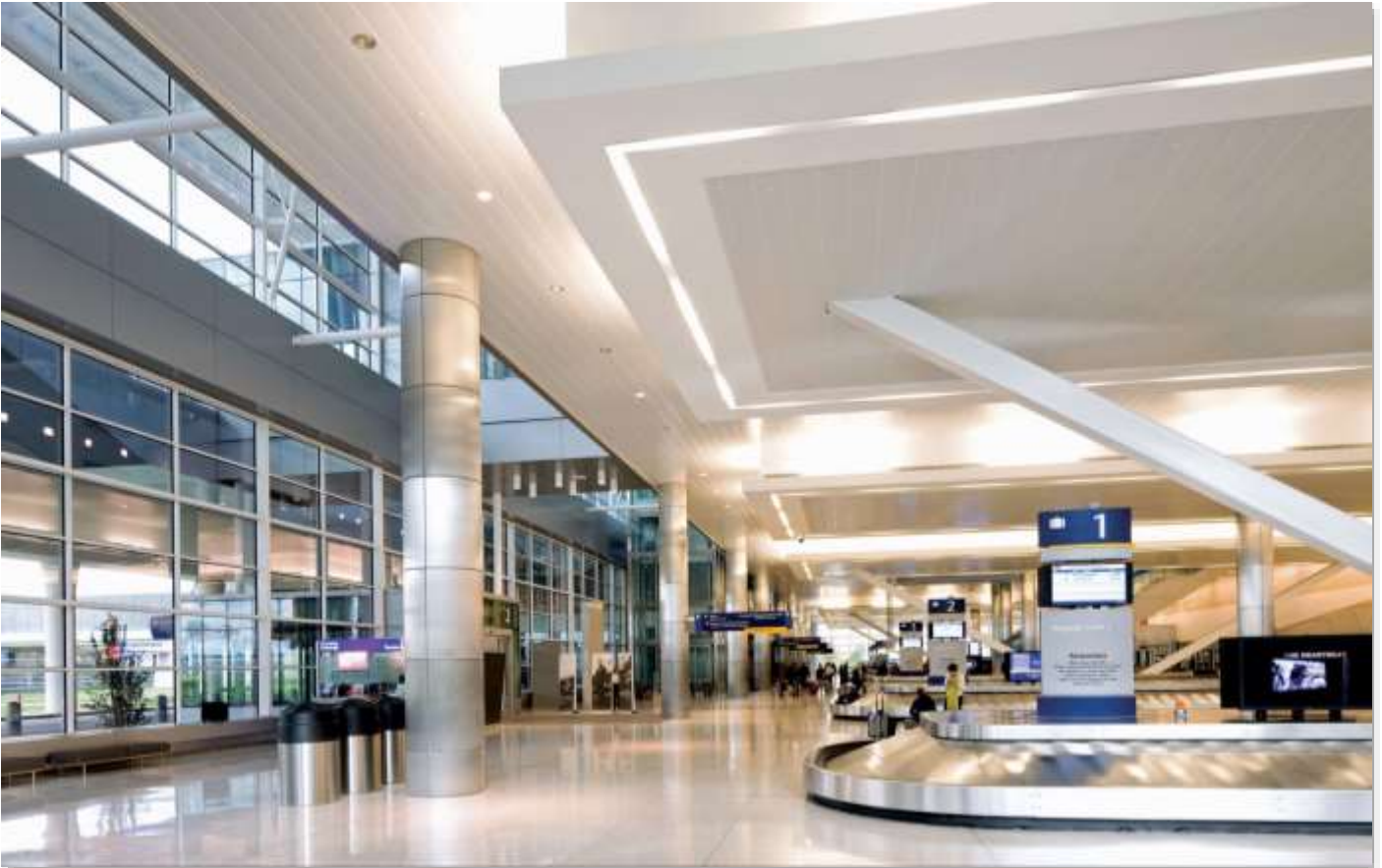
Figure 89: Indianapolis International Airport by HOK - Example of Sloped Baggage Carousel and Baggage Claim Area
