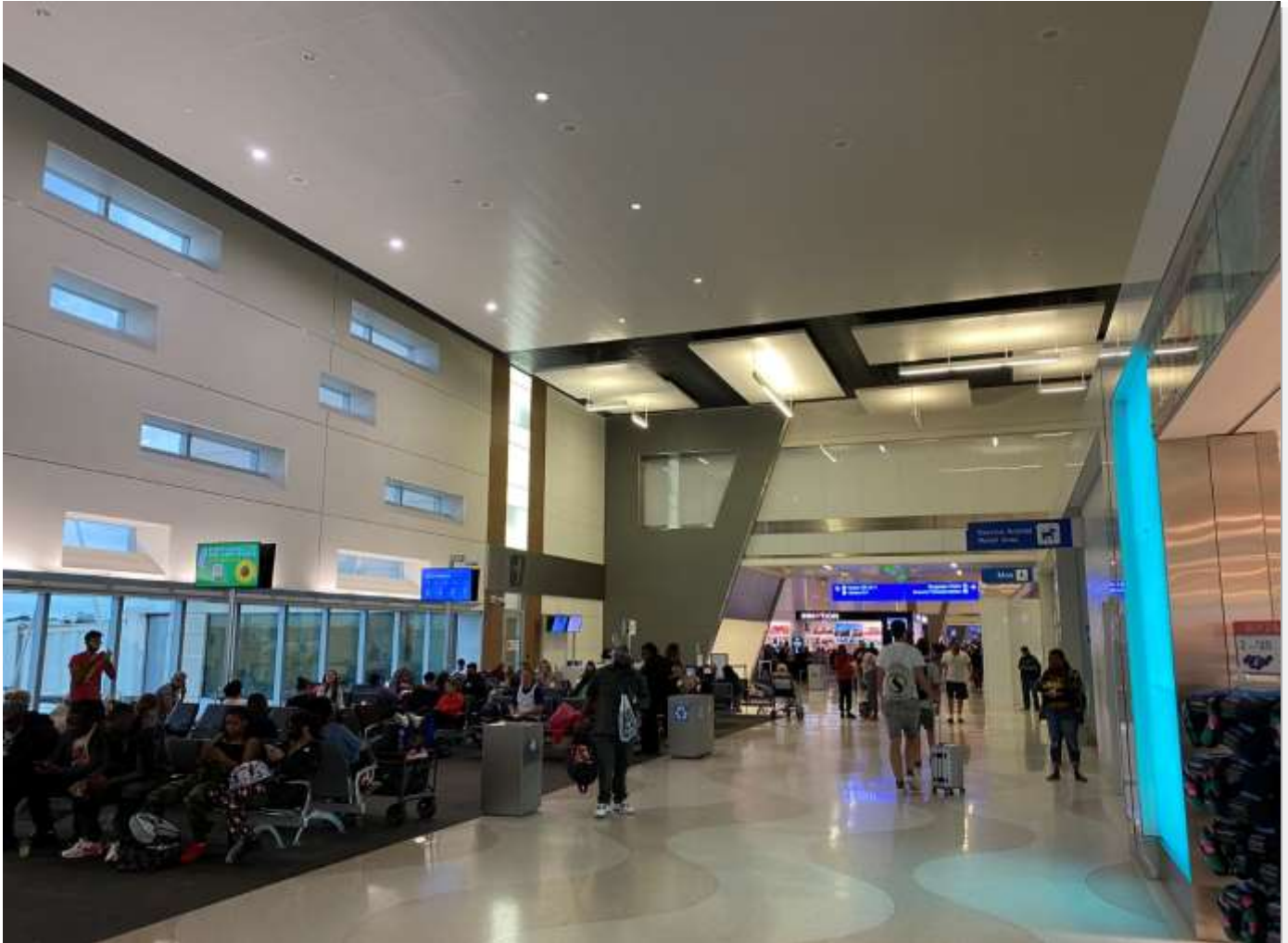
Figure 43: FLL Terminal 4 Concourse G Ceiling
