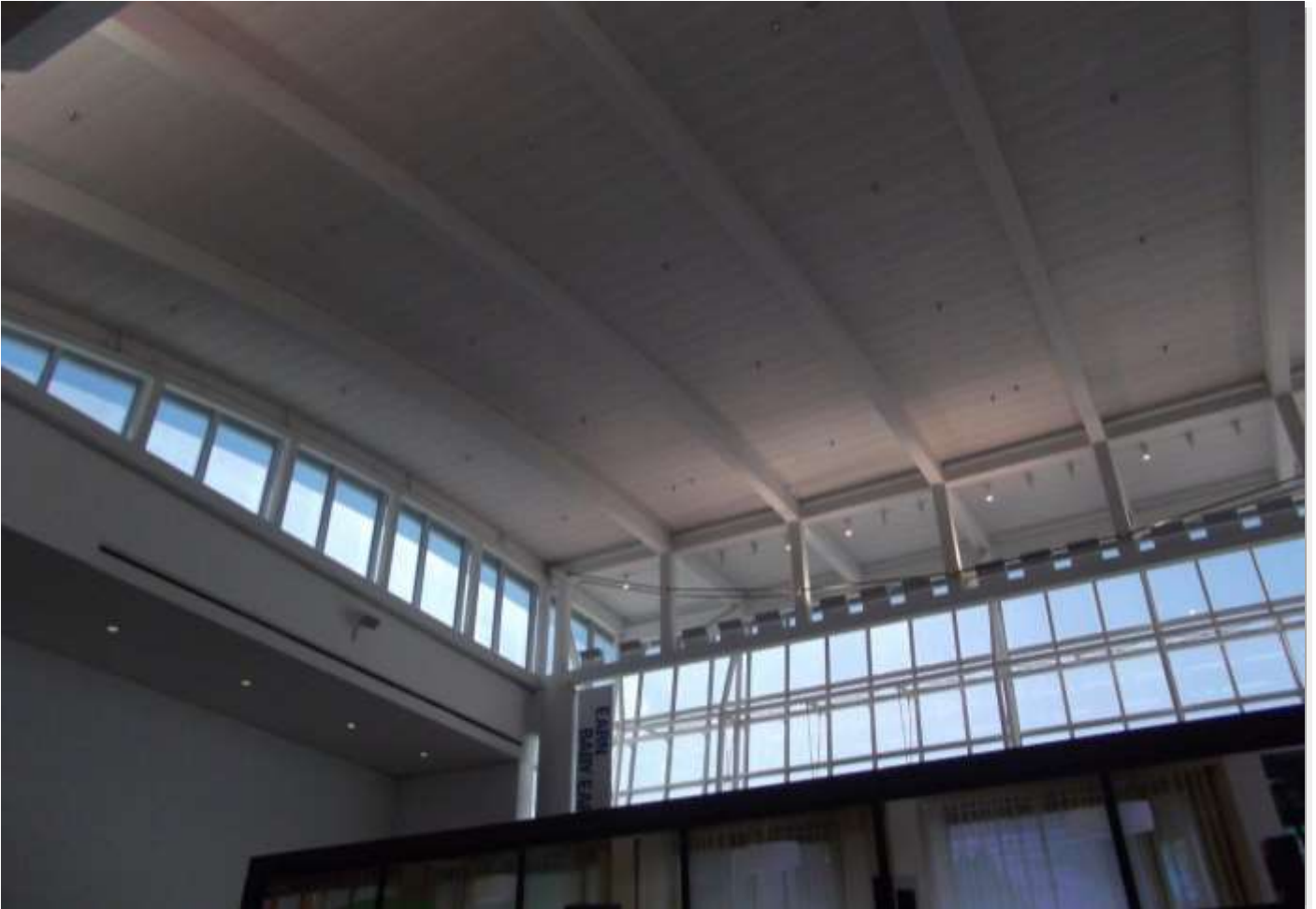
Figure 112: Example of Clearstory Lighting
