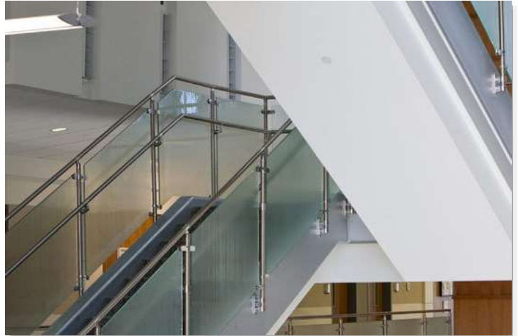
Figure 54: Frosted Glass Inserts on a Stairway Rail
