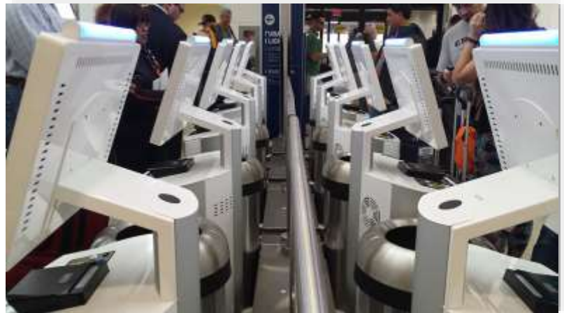
Figure 70: Example of existing FLL E-ticketing Kiosks connected in series to a bank.
