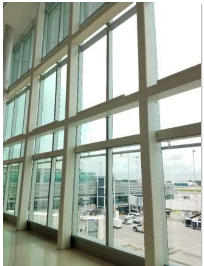
Figure 21: Curtain Wall Glass System at FLL T1 B/C Connector
