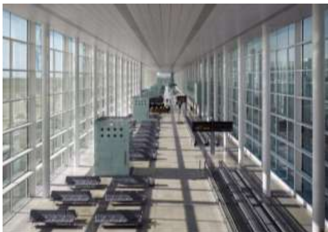
Figure 22: Detroit International Airport Concourse Glazing
