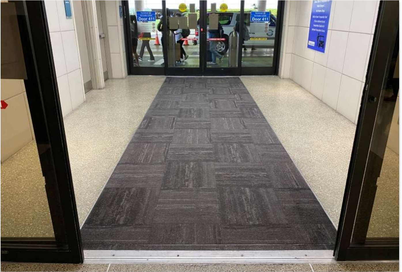
Figure 33: Existing FLL Terminal Vestibule Entrance Flooring
