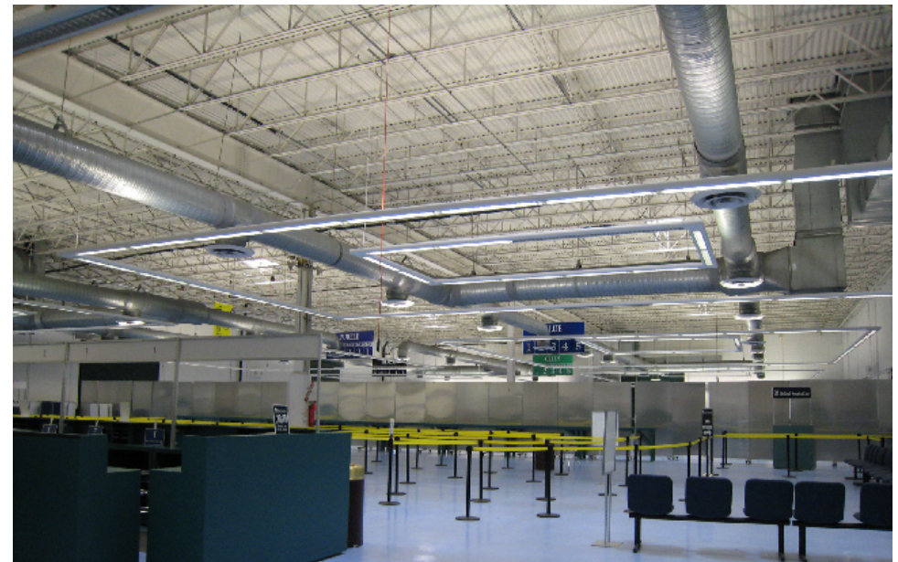
Interior View with Aluminum Barrier Walls
