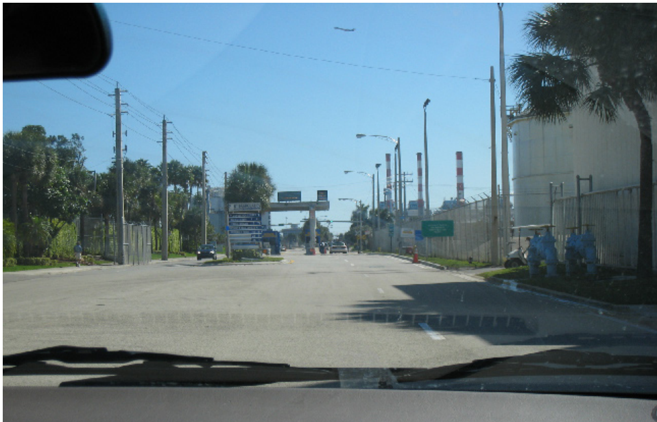
View of Eisenhower Boulevard to Security Gates
