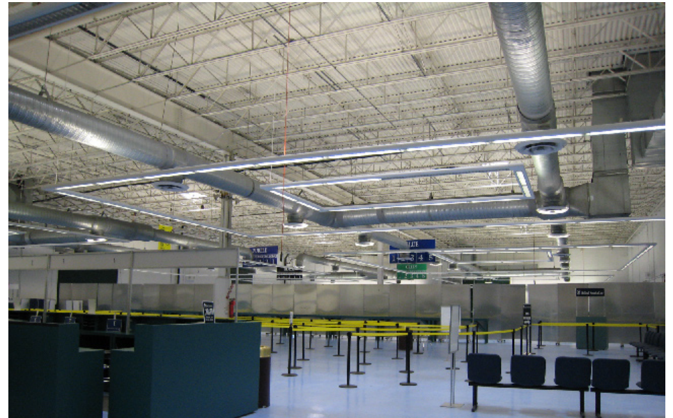
Interior View with Aluminum Barrier Walls
