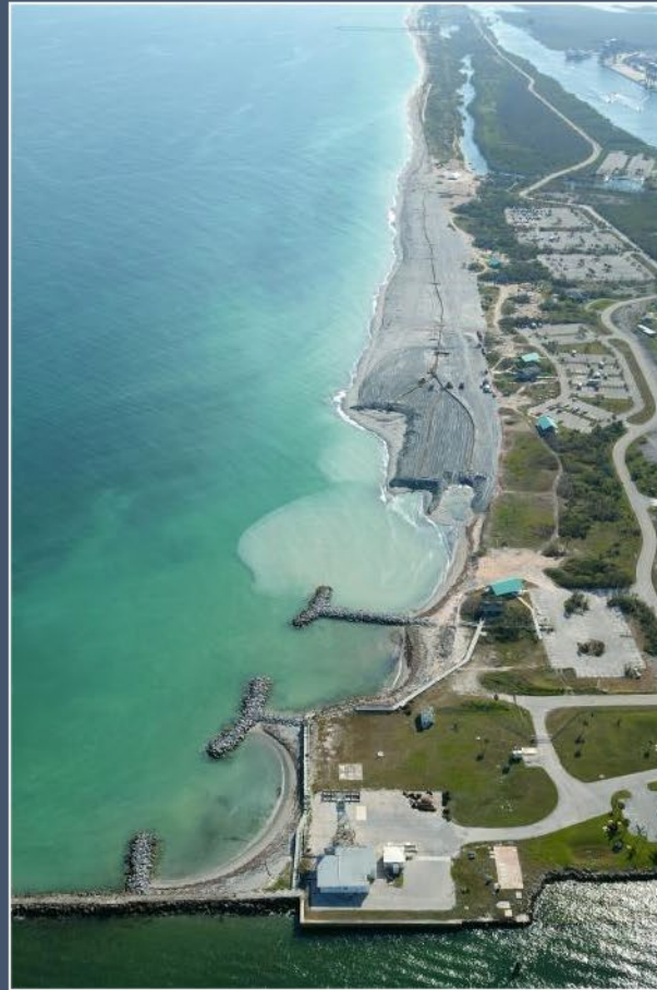
January 4, 2006 In Progress
