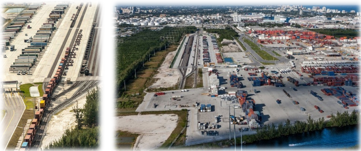
The 42.5 acre ICTF (Policy P1.1.5) consists of approximately 21,000 feet of track. Prior to its development, containers had to be conveyed to and from the Port to off-port rail terminals located on Andrews Ave.
