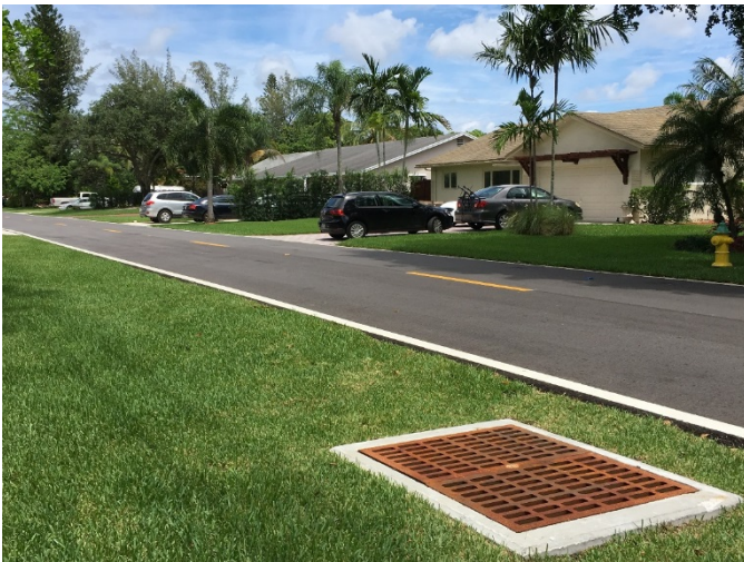
Hillsboro Pines Neighborhood Project improvements include stormwater drainage sanitary sewers, lift station and street enhancements.
