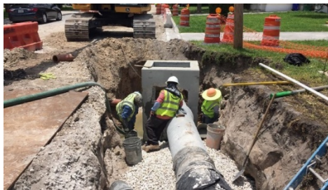
Drainage improvement project completed in Washington Park
