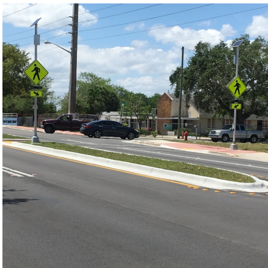
BMSD Safe Streets Project – Phase I : landscaped medians, decorative crosswalks with flashing beacon and bike lanes from NW 24 Ave and 6 Street (Sistrunk Blvd) – pictured- down to 27 Avenue
