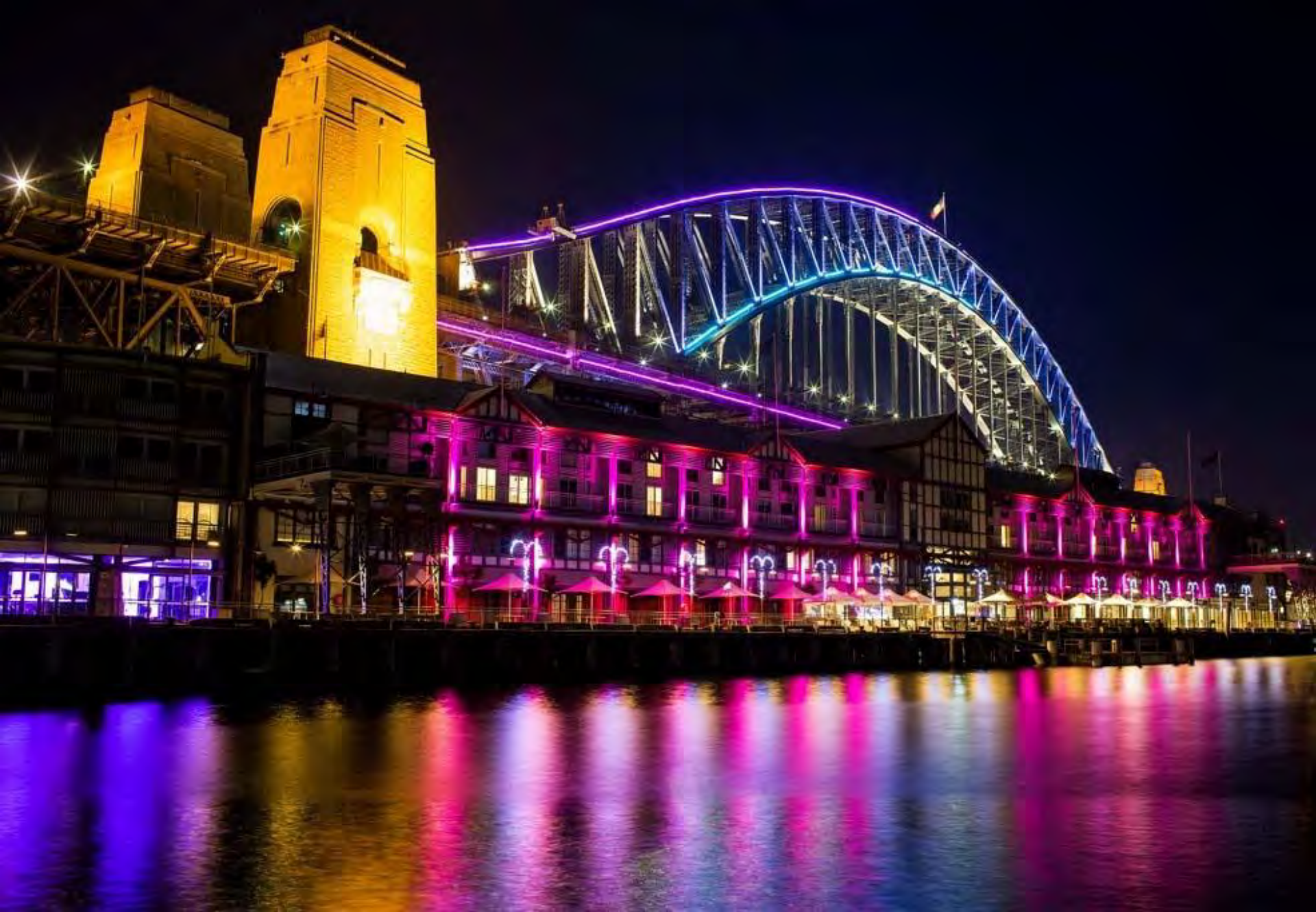
Bridge as a Gateway - Sydney Darling Harbour
