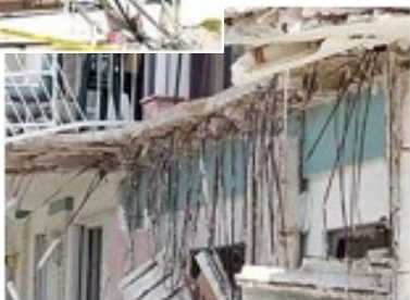
(Above, Right) A 1996 balcony collapse at 4111 S. Ocean Dr., Hollywood, FL
