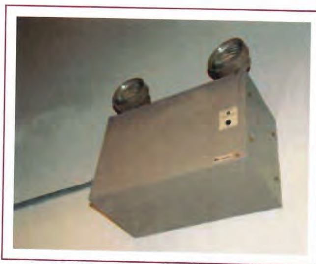
EXHIBIT 700.8 Self-contained, fully automatic unit equipment for operating emergency lighting located on the unit or for remotely located exit signs or lighting heads. (Courtesy of the International Association of Electrical Inspectors)
