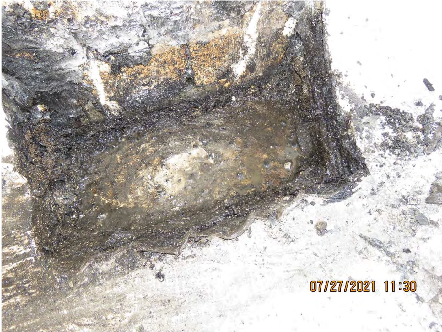
This photograph shows a roof section cut at the parapet wall and the clearly saturated conditions
