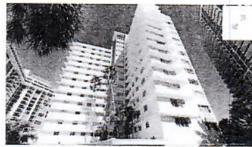
Carlton Terrace at 10245 Collins Ave., Bal Harbour.
