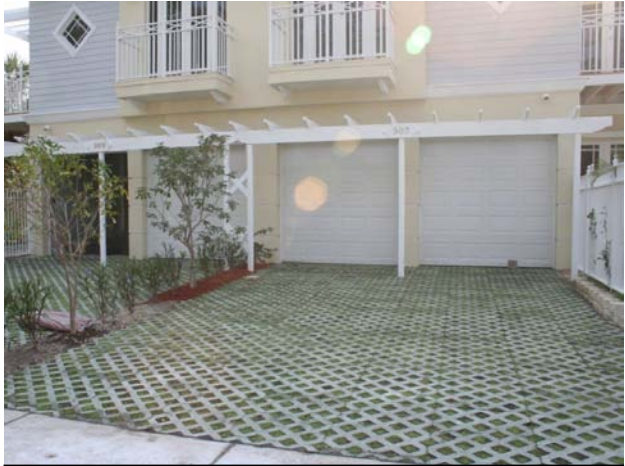
This driveway is pervious. It prevents stormwater runoff by allowing water to percolate and recharge the aquifer.
