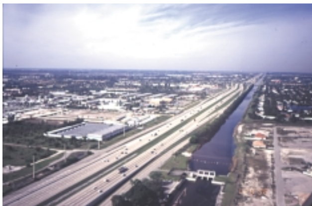
North New River Canal at Sewell Lock and Interstate 595, east-central Broward County.
