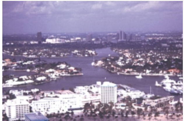
Confluence Intracoastal Waterway and New River, Ft. Lauderdale, eastern Broward County.
