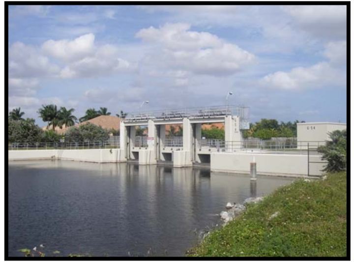
South Florida Water Management District G54 at east end of freshwater North New River Canal (view is to northeast)
