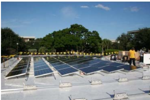
JM Family Enterprises Solar Project
