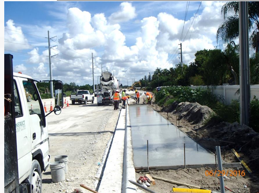
Proposed Sidewalk Construction
